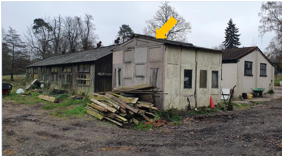
Photo 1: The existing barn (to be demolished)
