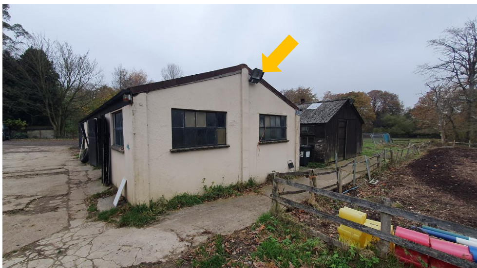
Photo 2. Existing stable - East elevation
