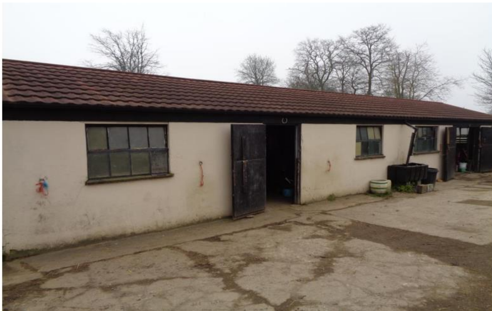
Photo 1. Existing stable (Conversion and re-use) – South elevation.
